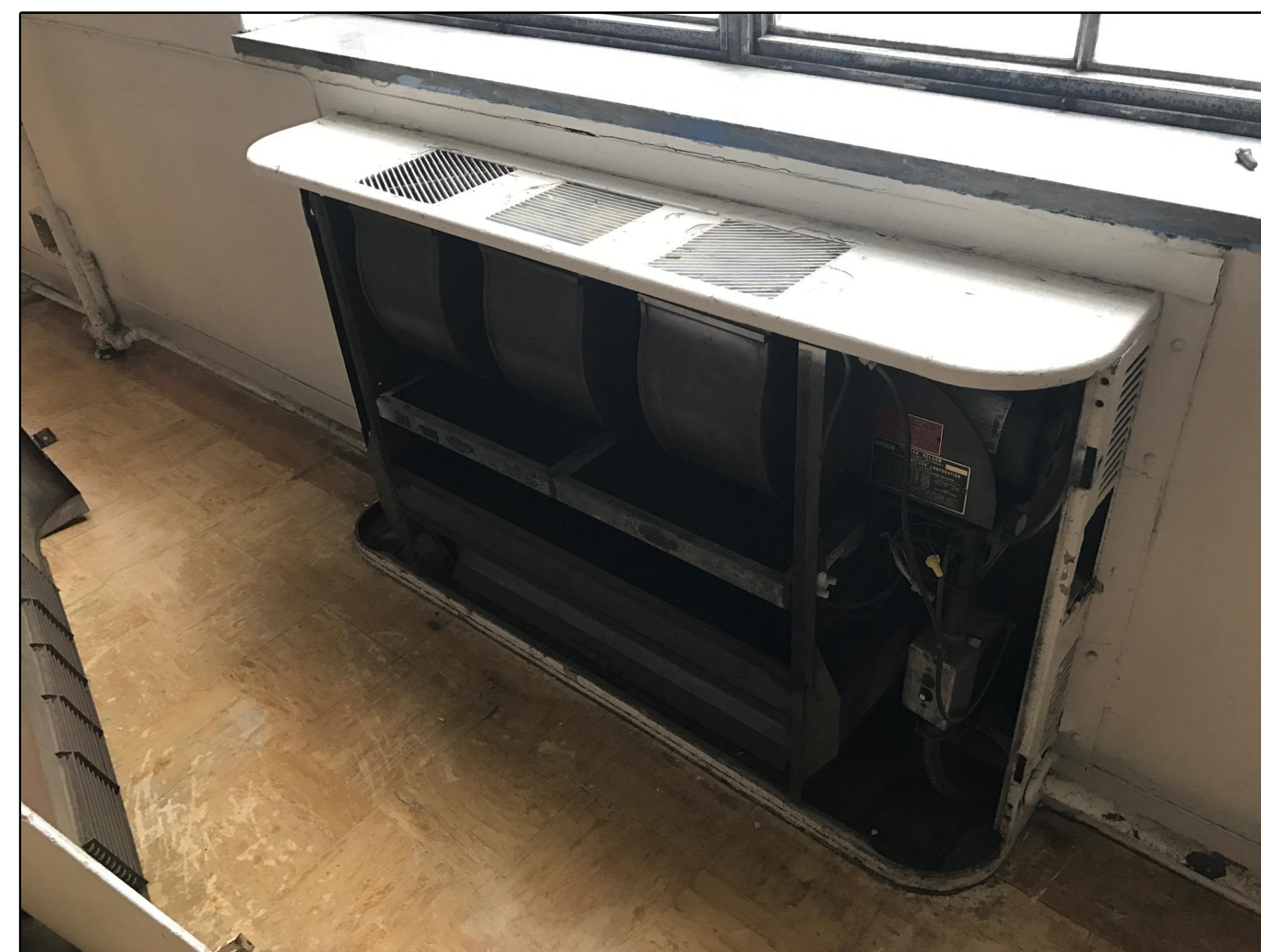
EXISTING UNIT VENTILATOR - TYPICAL
