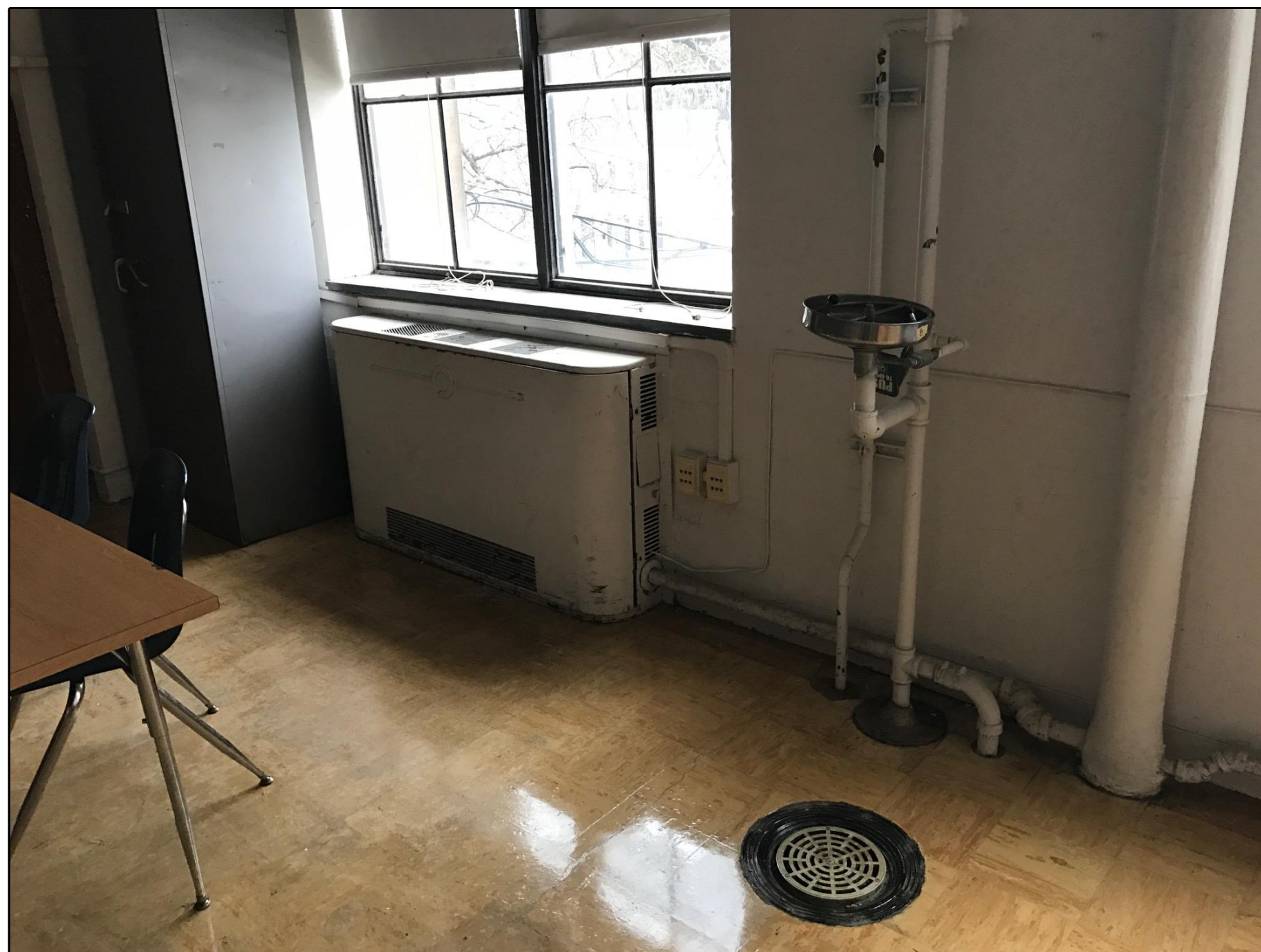
EXISTING UNIT VENTILATOR - TYPICAL
