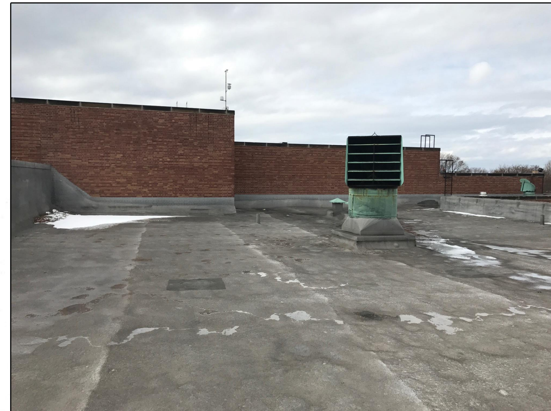
FLAT ROOF AREA FOR EXTERIOR MECHANICAL EQUIPMENT
